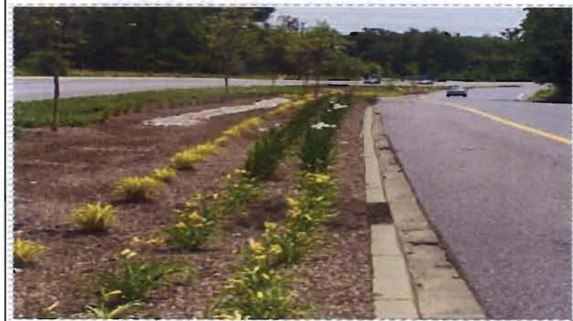
Figure 5.1. Bioretention cell in Adelphi Road median, Adelphi, MD. Note curb cuts for water entry.
