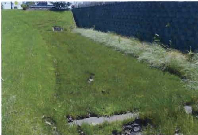
Biofiltration Swale With Spreader Bar on SR 503 in Clark County.
